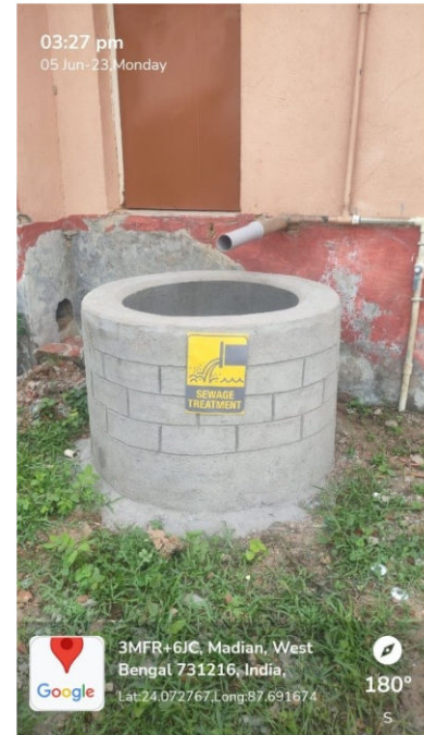
Fig 7.3: Liquid waste pit
