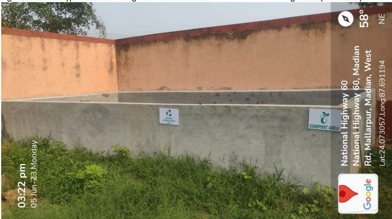
Fig 7.4: Composting Area for Biodegradable waste
